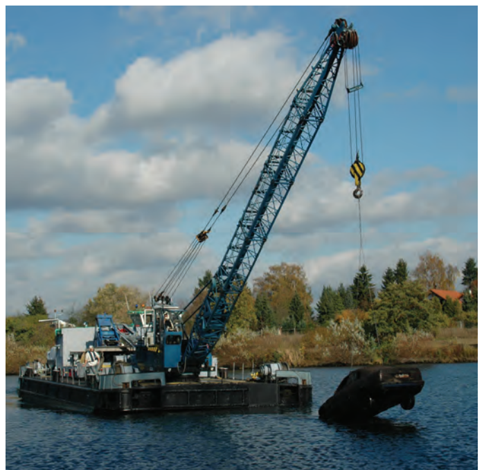
Securing of evidence following UPEX® sounding
