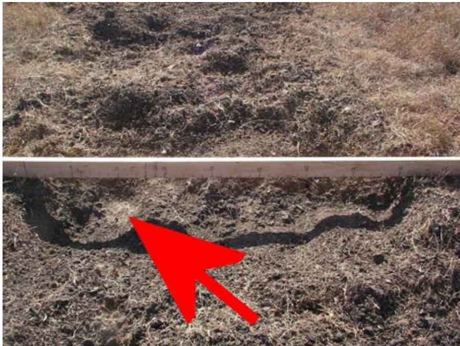
Figure 15. Deep Hammer Penetration in Soft Holes
