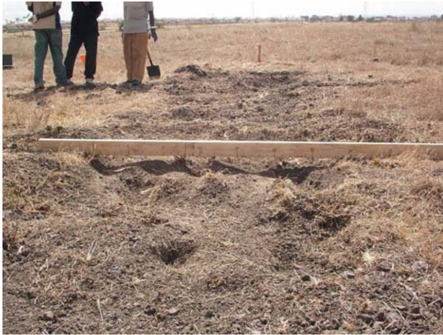
Figure 14. Poor hammer penetration in hard surface
